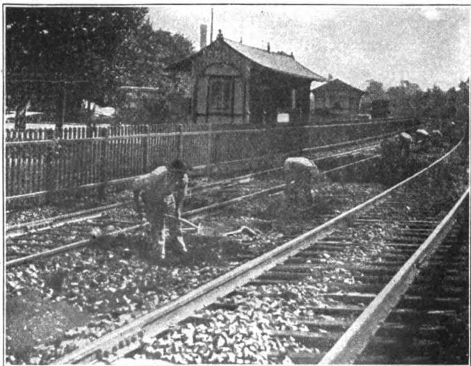
Fig. 8. Forking and Cleaning Stone Ballast.
