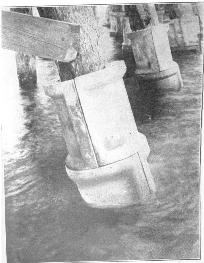
Lock Joint Pipe on Batter Piles.
