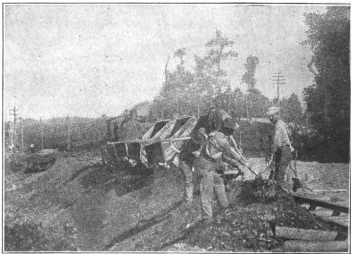
Fig. 67. Widening Embankment.
