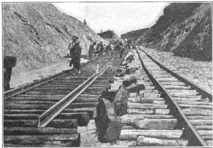
Fig. 51. Laying Track.
