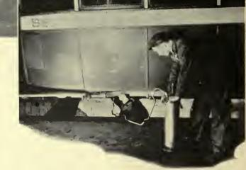
Power generators and motors are lubricated with a special ball-bearing grease
