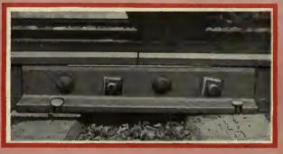
The above shows Joint Shim in position between Bar and Ball of Rail.
