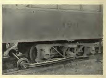
Dolly used by Cincinnati Street Railway to bring in car with broken axle
