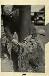
Shaping the cement cap over top of OB Pole Sleeve to shed water and moisture.
