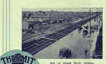
Job on Grand River Avenne, Detroit, completed with standard steel tie and Thermit welded joint construction.
