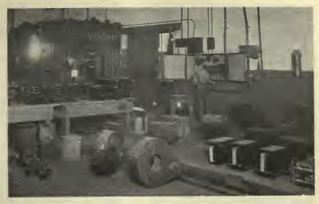
Section of the electrical equipment department where line breakers, circuit breakers, lightning arresters and other apparatus are overhauled
