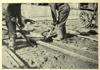
Pneumatic hammers with block tool points were used to drive the concrete thoroughly to place in the foundation
