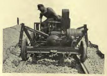
Track was brought to correct line and grade by machine tamping
