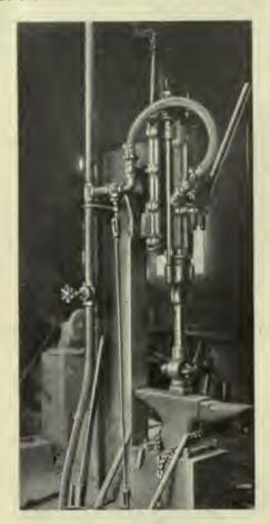
Air hammer made from an old rock drill speeds up blacksmith work in the track department of the Georgia Power Company
