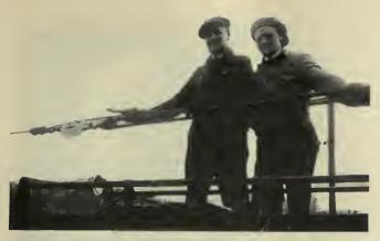
Measuring the trolley wire tension with a dynamometer
