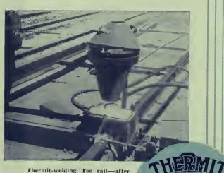
Thermit-welding Tee rail—after reaction has taken place, but before removing moulds.
