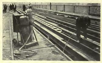
Portable truck for oxyacetylene burning outfit used by the Cleveland Railway
