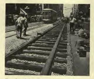
Treated wood tie and stone balast sub-structure is used to serve through the life of two rails in Memphis
