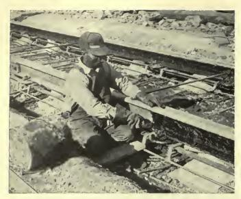
The rail is coated with about ¼ in. of plastic asphalt material applied with a paddle as shown
