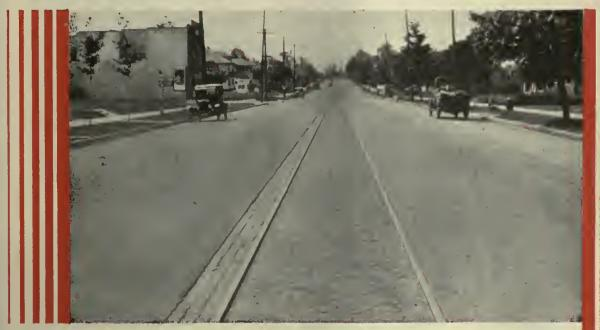
The track shown above is a continuation of the track shown in picture No. 1, opposite page. But in this section Dayton Ties were used. Note the unbroken pavement and absence of any sign of "VIBROLITION."
