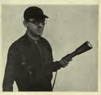
Inspection light used by Cleveland Railway has electrically heated handle
