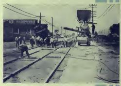
Same job, showing method of concreting using two mixers simultaneously on opposite sides.
