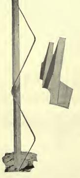
Four of the expanded angles shown above make one pole, including all lattice members.
