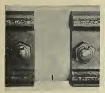
The standard practice of undercutting rails from head to foot permits a gap to appear as the rail wears which gradually causes cupping
