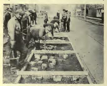
When paving with granite blocks the Cleveland Railway uses straight edges to insure level surface
