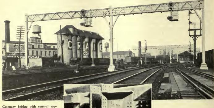
Catenary bridge with central supporting member, showing also the new signal installation
