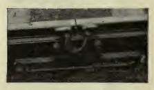
Close-up of O-B Titon Bond installed on track of above property.
