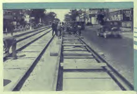
Reconstruction work in Jefferson Ave., Detroit, 2200 feet of new track laid and Thermit-welded beside the old without stopping ears.
