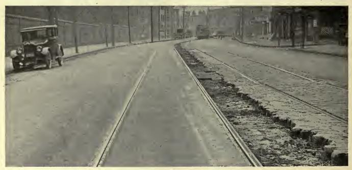
The paving surface consists of a 3-in. layer of sheet asphalt
