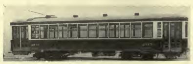
The lighter metal was first used in Canada by the Montreal Tramways. total of 80 cars with aluminum are now in service on this property
