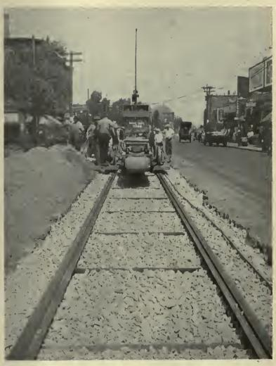
Mixing apparatus mounted on railway trucks was used for grouting
