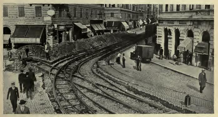
While new trackwork was installed service was continued uninterrupted over old track
