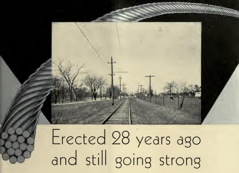
This feeder cable, erected 28 years ago by the Columbus, Delaware and Marion Electric Company, is a striking example of the reliability of aluminum cable.
