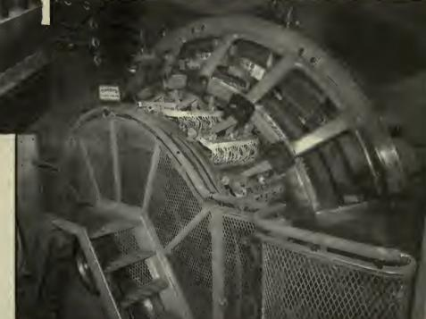
Above. An Edison 250-light type K generator in use from 1883 to 1928. Equipped with copper leaf brushes.
