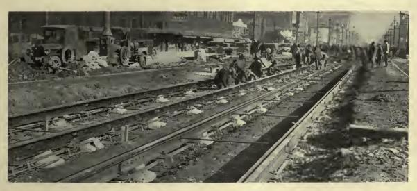
Rails in position with the anchorages attached and clips tightened. Wooden wedge blocks are used on top of pedestals to obtain surface grade adjustment
