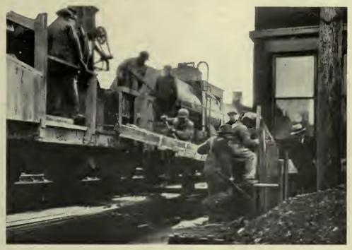
Pouring concrete for a signal bridge foundation under difficulties. By the use of a concrete train no space for installing mixing machinery was needed
