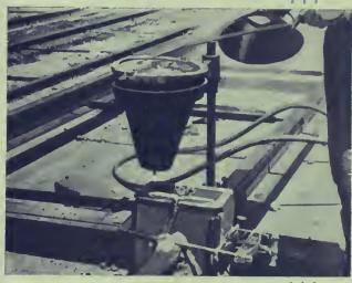
Thermit-welding Tee rail—showing crucible in place, with charge.
