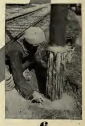
Cementing the base. Sidewalk poles are cemented flush with pavement.
