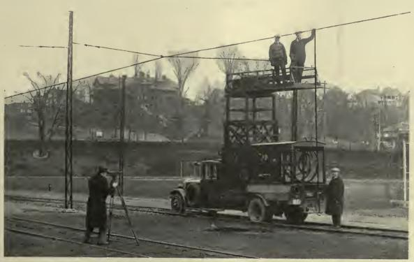
Checking up on tension of the trolley wire by measurement of the sag with a level
