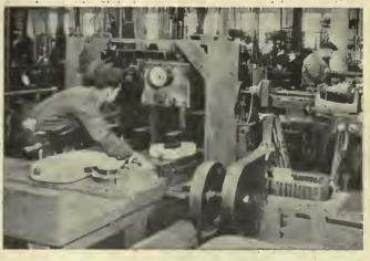
Field coil testing device and taping machine used in Cold Springs shop of the International Railway, Buffalo, N. Y.
