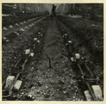
After the trench is graded, precast concrete pedestals are placed in position. The steel framework, made up in 20-ft. sections with anchorages attached, is then placed in position over the pedestals
