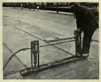
Vibration treatment compacted the concrete to an extent that required the use of 7 per cent more material than had been estimated
