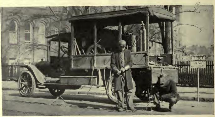
A complete electric welding set and an oxy-acetylene cutting equipment are mounted together on a 1-ton White truck by the Georgia Power Company
