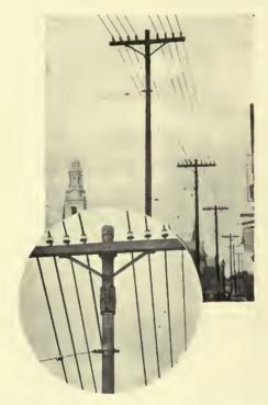
Pole height increased by clamping short extension to top of existing pole
