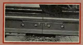
The above shows Joint Shim in position with angle bar removed.
