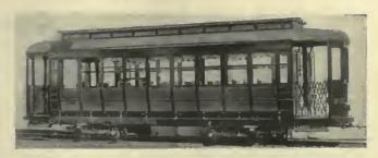
From the vintage of 1905—a car for Manila, using aluminum to withstand the ravages of "white ants"
