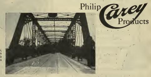
Spy Run Bridge, Ft. Wayne, Indiana, smooth-surfaced with Carey Elastite Asphalt Plank. Notice also that the rails are cushioned with Carey Elastite System of Track Insulation.
