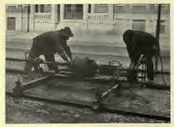
Penetration of the grout was assured by use of a revolving vibrator placed longitudinally between the rails
