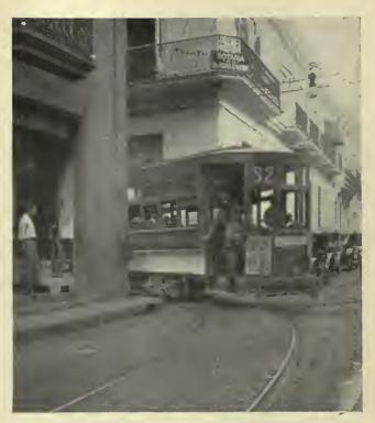
Single-truck cars and sharp curves are typical of electric railway operation in Havana
