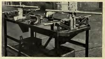
Portable bench for reaming and finishing relined bearings in the Hamburg Elevated Railway shops
